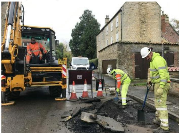
After a series of flood events in the village, it's clear the brick Roman and Victorian drains no longer do the job. Highways have spent some weeks digging up the road and replacing the drains. A huge thank you.
